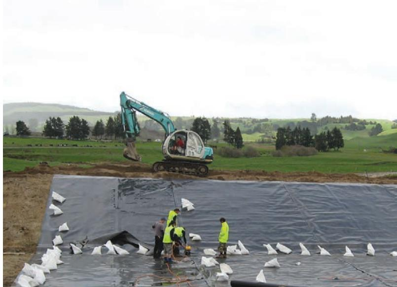
Storage pond for dairy shed effluent allowing land based effluent application at optimal times.
