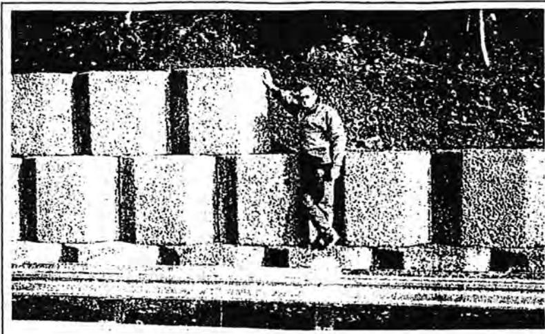
interlock area extends from the rear surface by a distance of 150 millimetres and serves to lock the block to blocks placed below. The rough exposed concrete surfaces of the block aid the resistance to shearing forces by increasing the friction between units.
