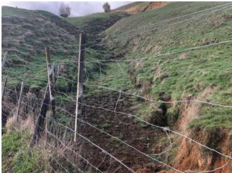
Sediment trap that is dry (no water flowing) because of drought
