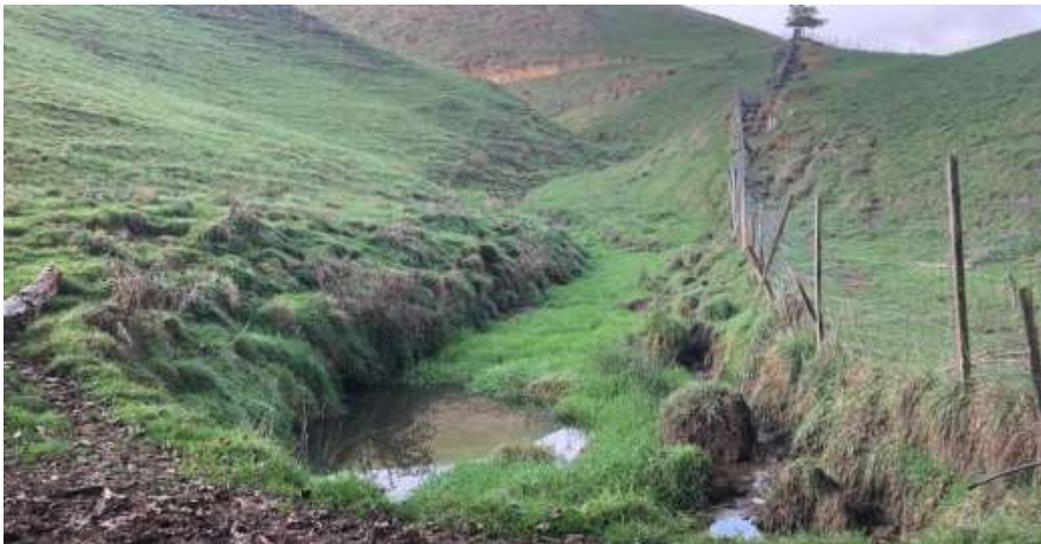
Sediment trap that has been in for 37 years and has been cleaned on two occasions over that time
