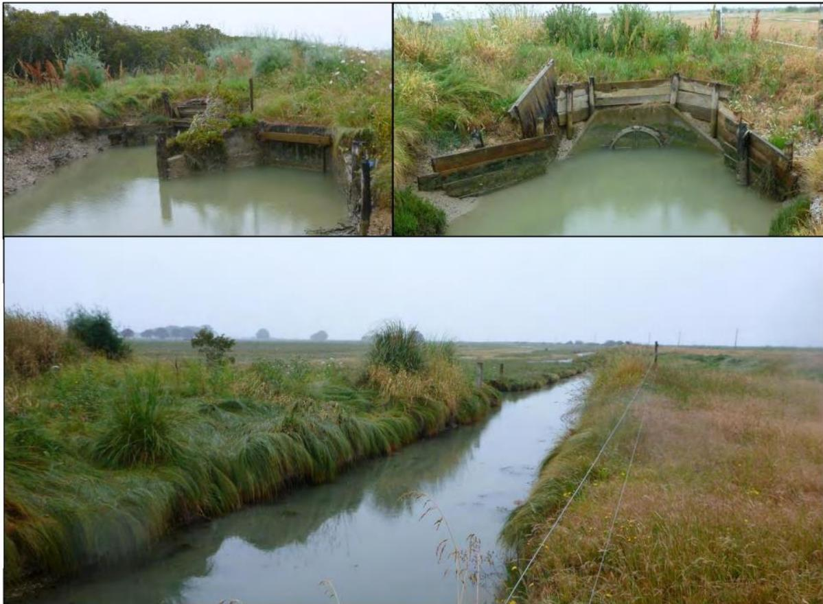
**Figure 14** Existing flood control gates and Pūkoro Stream upstream of the gates. Photos were taken on an incoming tide. Note mangroves in the Miranda Stream (top left photo) (Franklin District Council, 2007, p.6).
