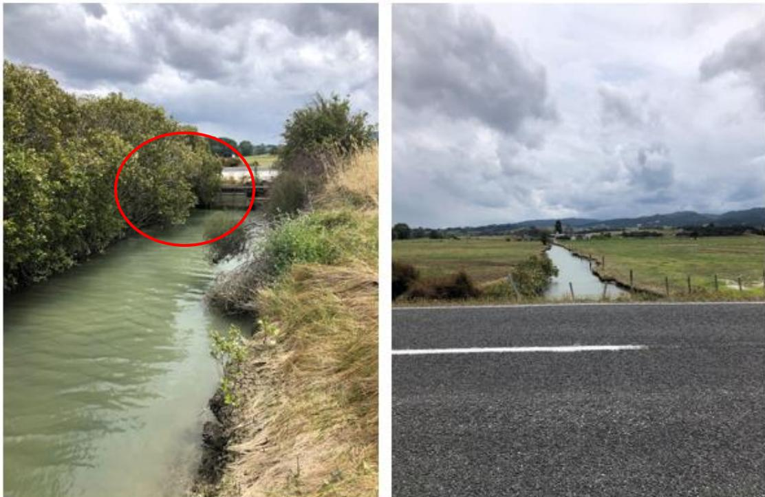
**Figure 13** Photos of a floodgate and culvert underneath ERC and a channel through rural land on an outgoing tide. Note you can see the misalignment of the metal floodgate with the culvert size allowing saltwater to pass through (Mills W, 2021b).
