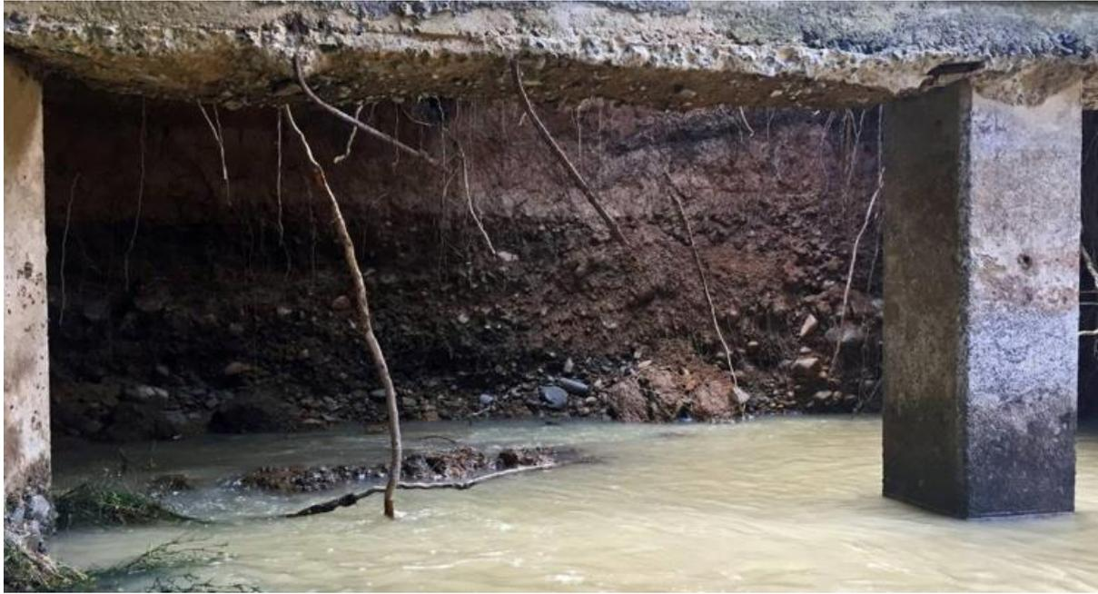
**Figure 11** Eroded bridge abutments at Waharau Bridge following Ex-Tropical Cyclone Debbie on the 4th - 6th April 2017 (Marsh et al., 2022, p.42)
