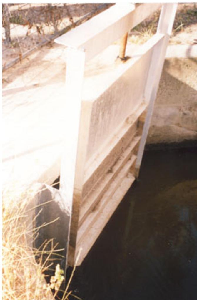
**Figure 11: Screening structure on inlet to Richardson's Lagoon**
