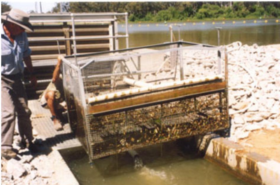
**Figure 4: Carp cage at top of Torrumbarry Weir fish pass**
