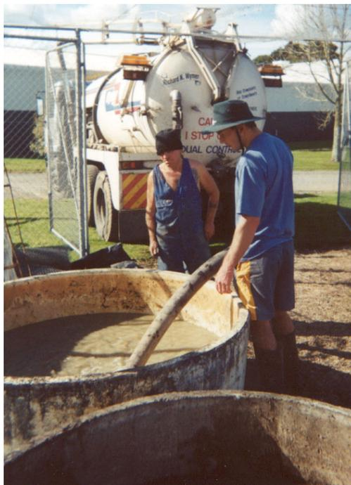
**Figure 4: Discharging sediment slurry into concrete troughs, 23 September 2003.**
