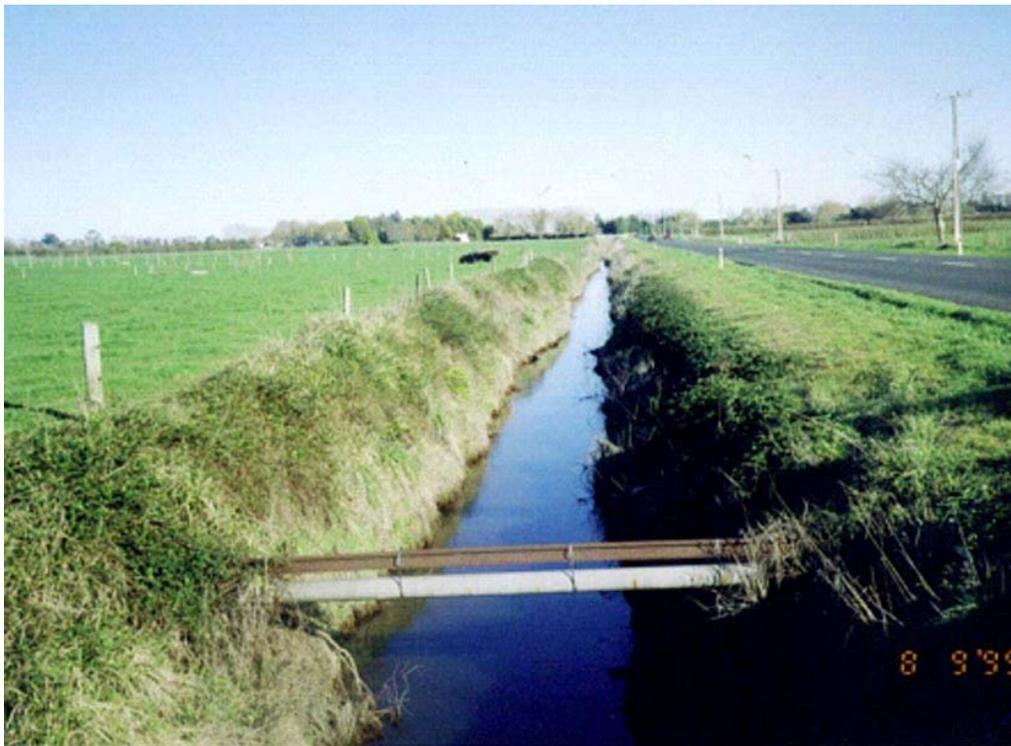
**Photo 6** The same drain as in photo 5 following fencing to exclude stock
