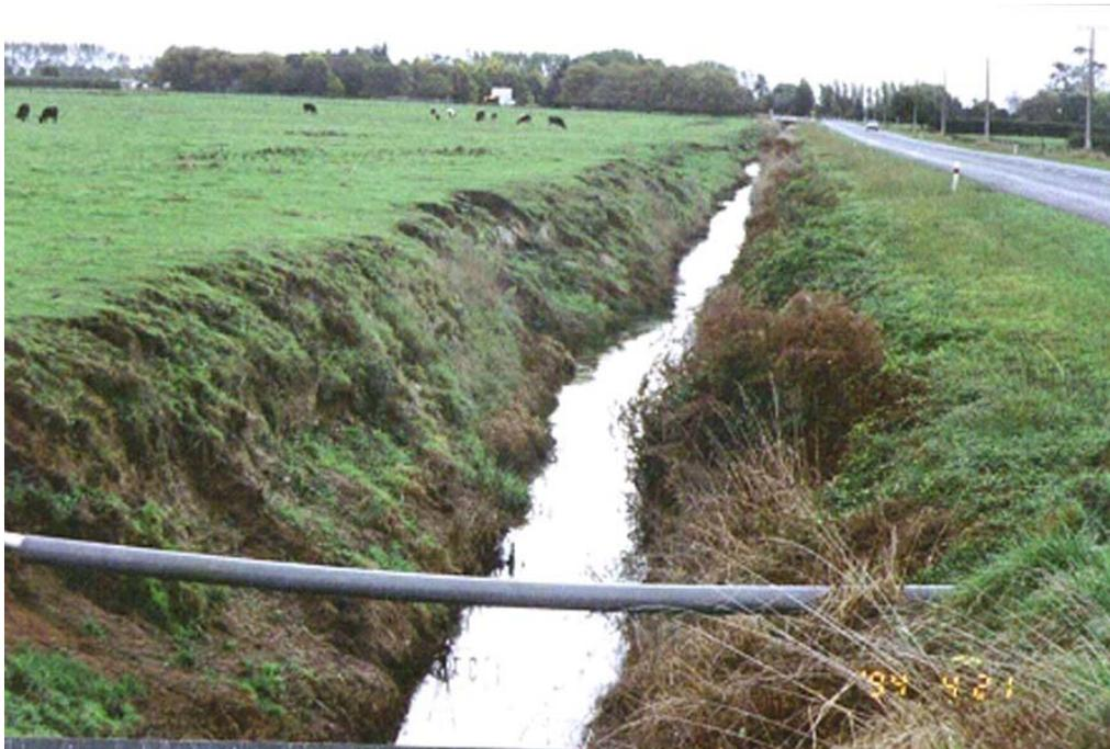
**Photo 5** Drain bank erosion caused by stock
