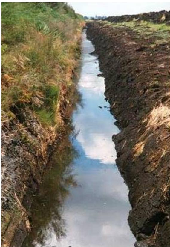
**Photo 12 Excessively dug drain**
