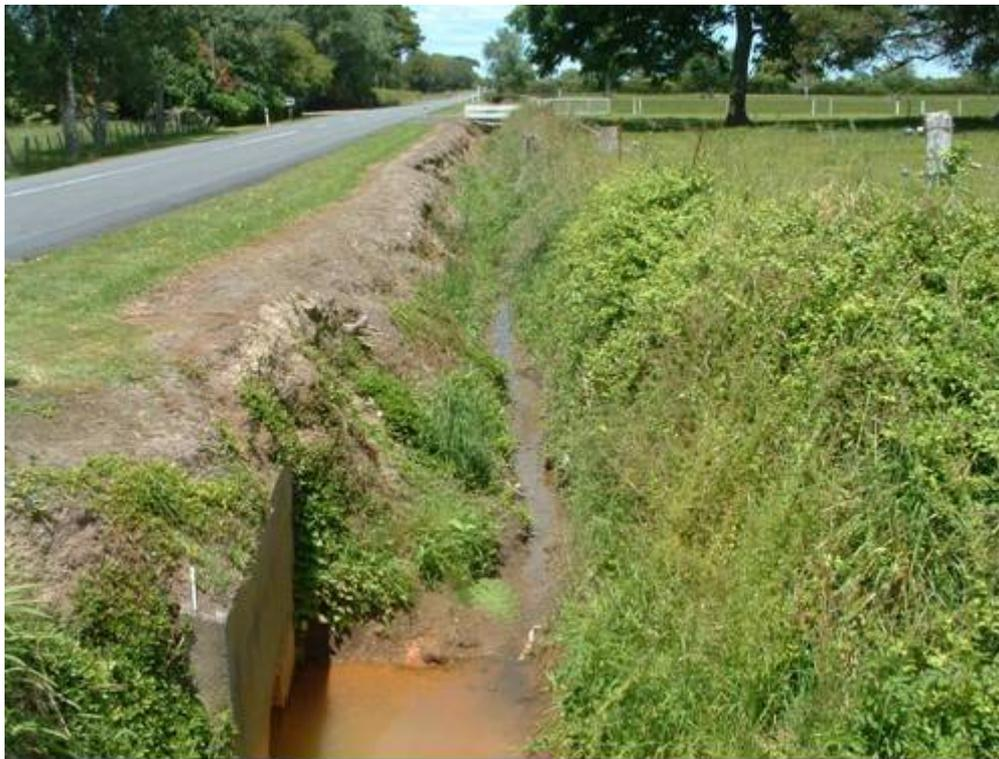
**Photo 9** Bank erosion resulting from spraying the drain edge. The proximity of the waterway to the road will result in storm water runoff and pollutants directly entering the waterway
