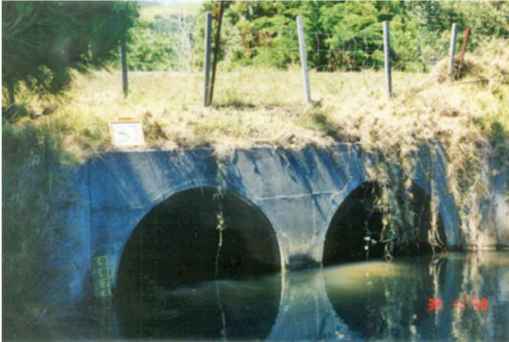
**Figure 7 Typical multi-barrel circular culvert**
