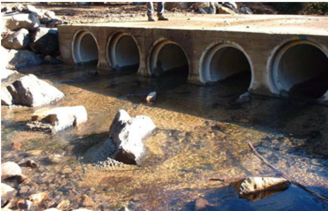
**Figure 8 Multi-barrel circular culvert with culvert pipes at different levels to cater for high flows**
