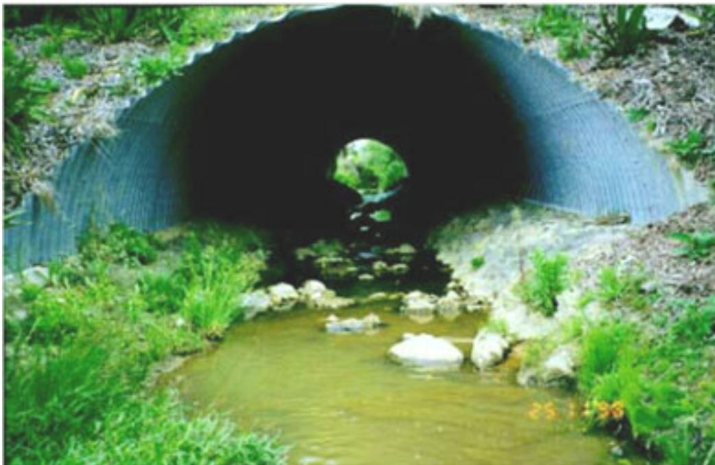
**Figure 3 Best Practice - single barrel arch culvert**
