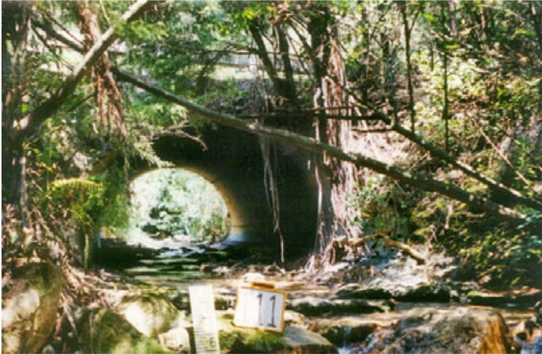
**Figure 2 Single barrel arch culvert**
