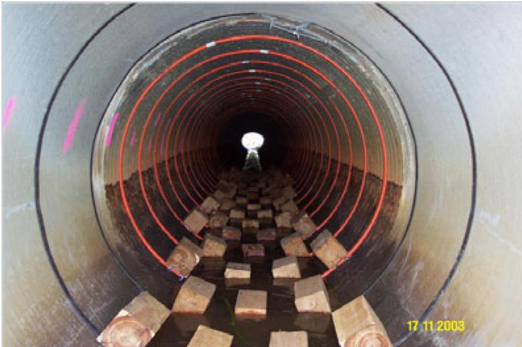
**Figure 10 Baffles (these can be of many materials) and rocks can be installed into the base of a waterway crossing to provide cover and low velocity zones to aid with fish passage**
