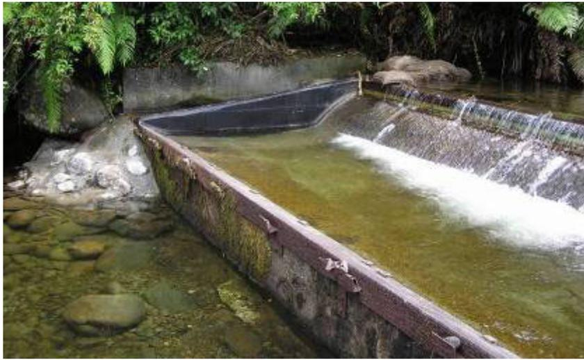
**Plate 14.** Weir structure at Mangauika Stream (Pirongia). Note the fish pass at the far bank.
