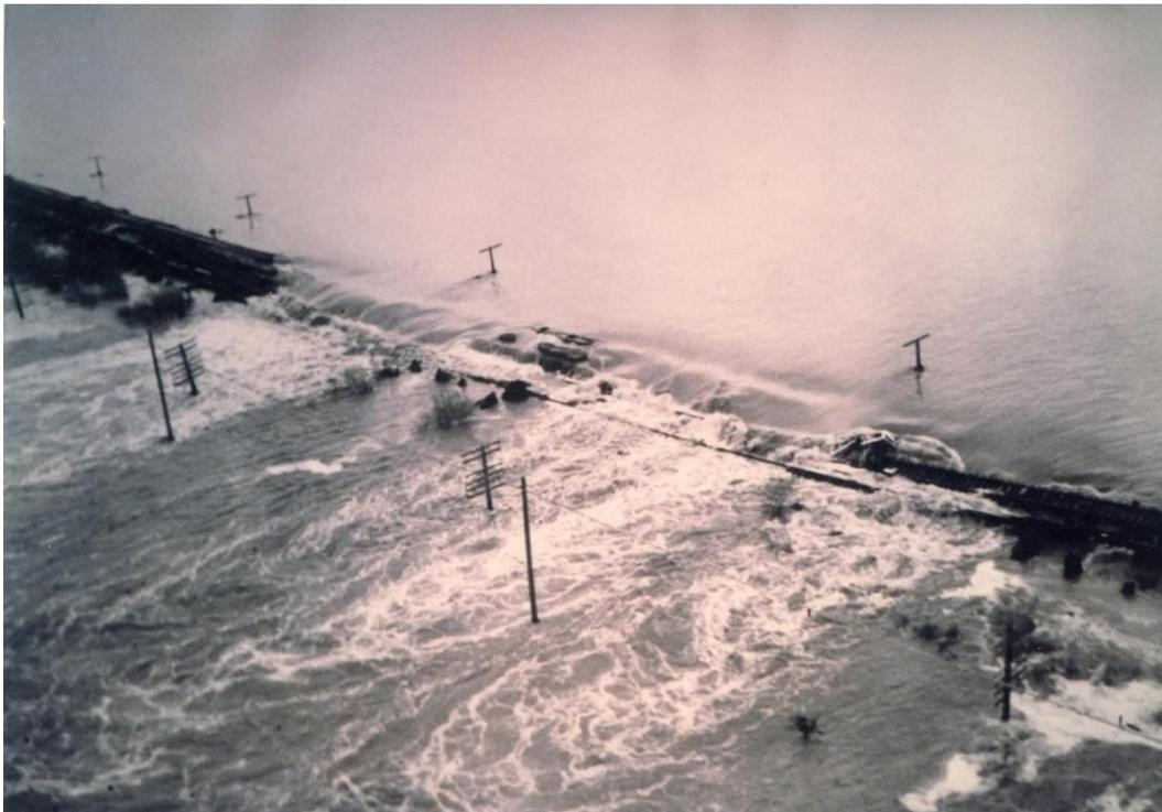
**Figure 12: Example of a stopbank being overtopped**
