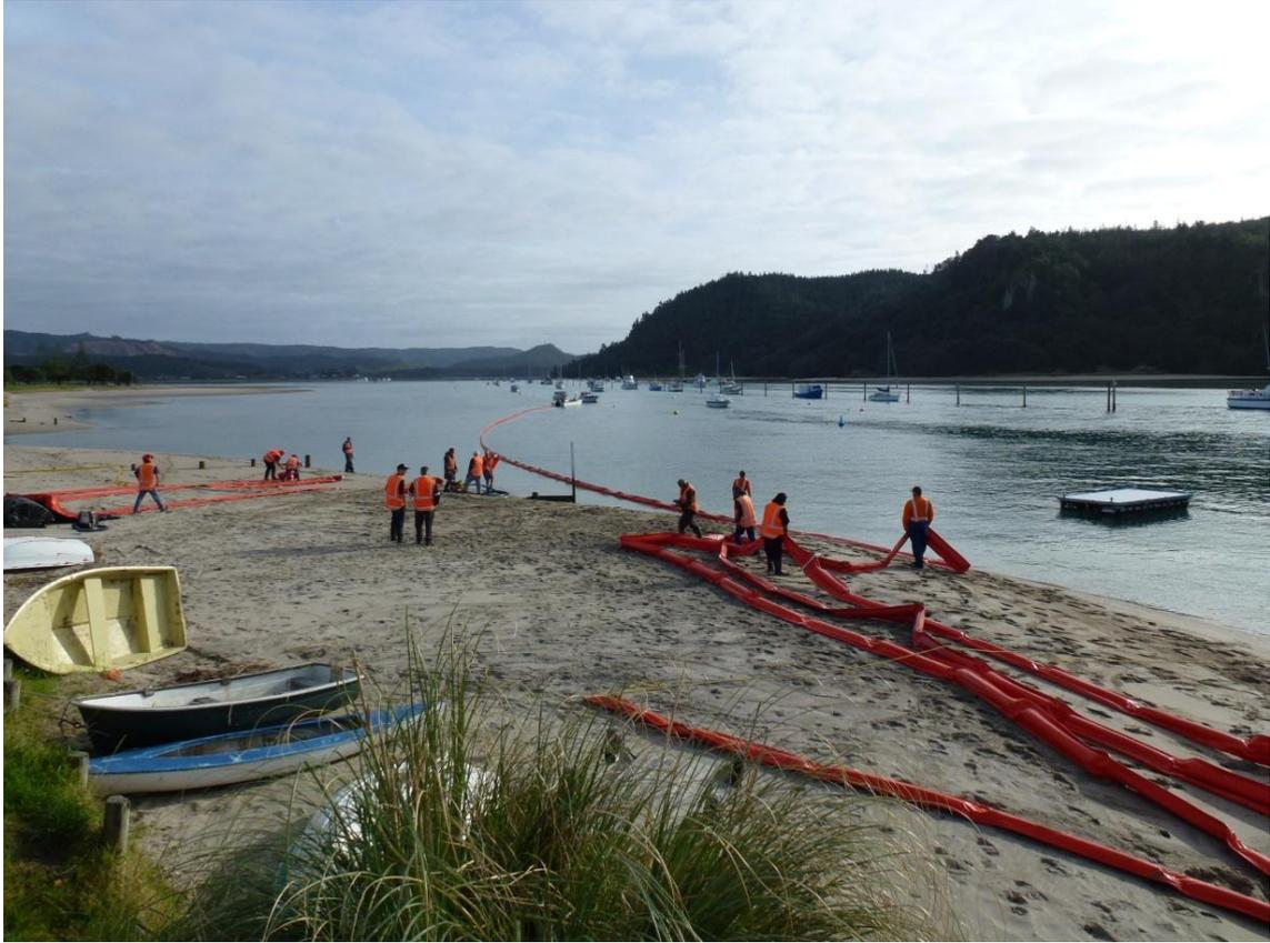
**Figure 5** Preparing booms for towing to set site
