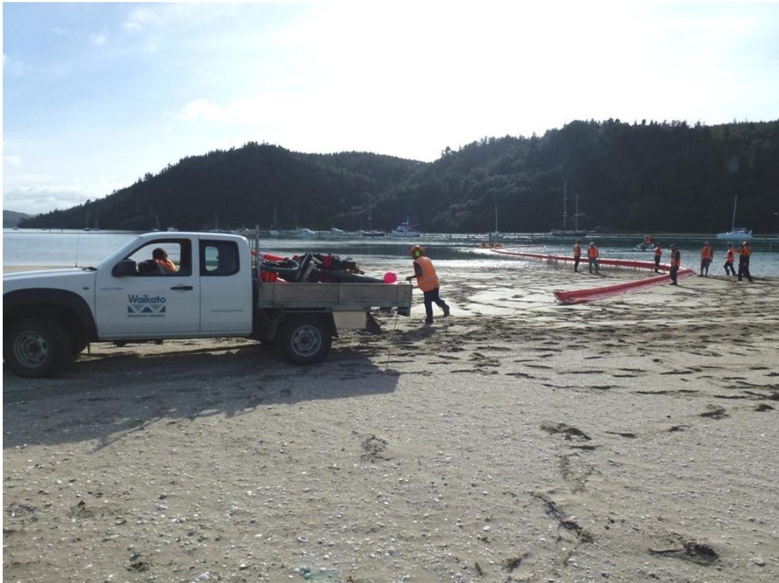
**Figure 8 Dragging the ballasted boom downstream**
