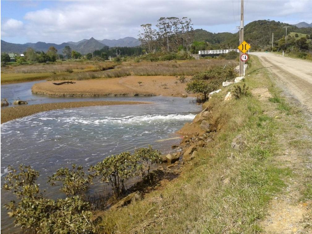
**Figure 11: A view of the constricted culvert under Kennedy Bay Road just north of Mangatu Stream.**
