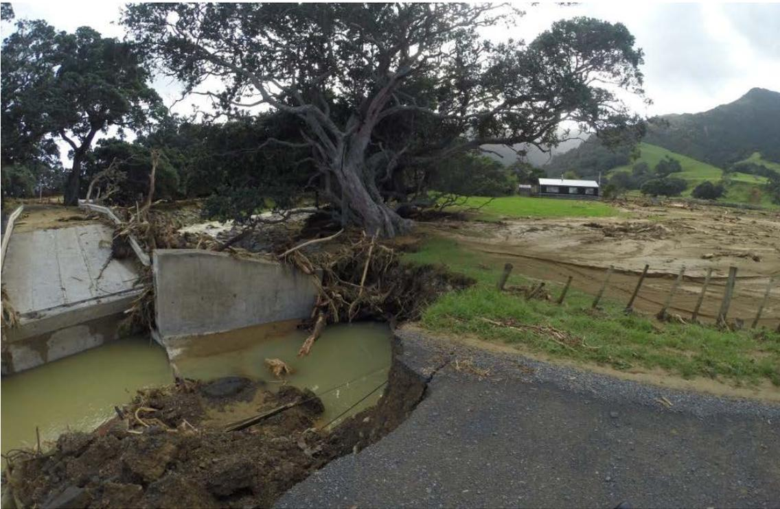
**Figure 13: - Ongohi stream bridge damage**
