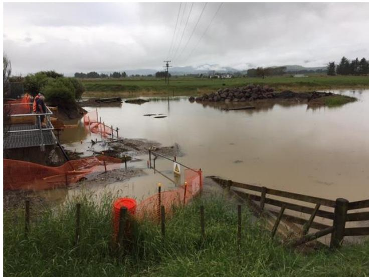
**Figure 17: Stocks Floodgate on 8 March showing coffer dam overtopping.**
