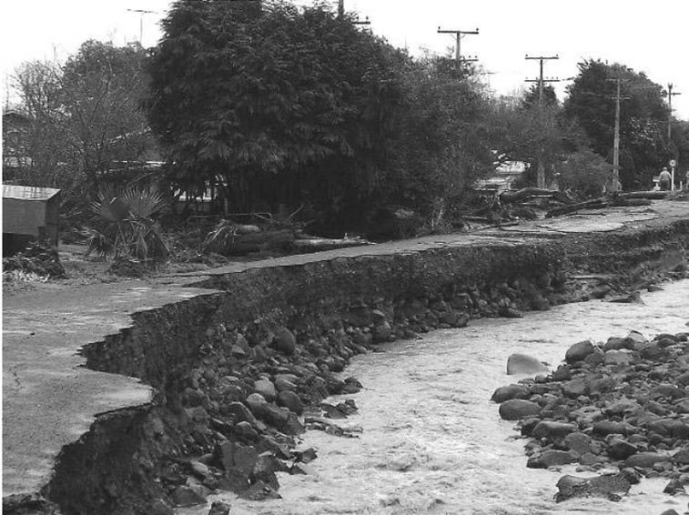
*Figure: Streambank erosion on Te Puru Creek Road during the 'weather bomb'*
