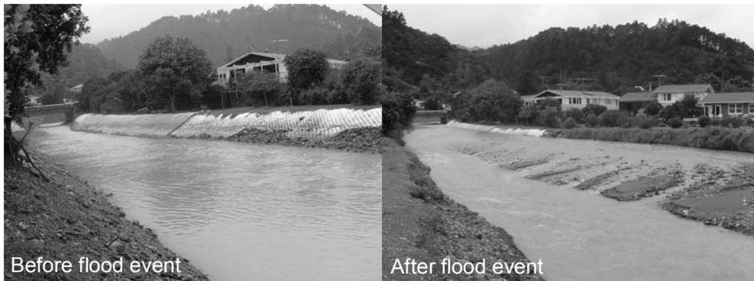
*Figure: Sedimentation in the Tararu Stream*
