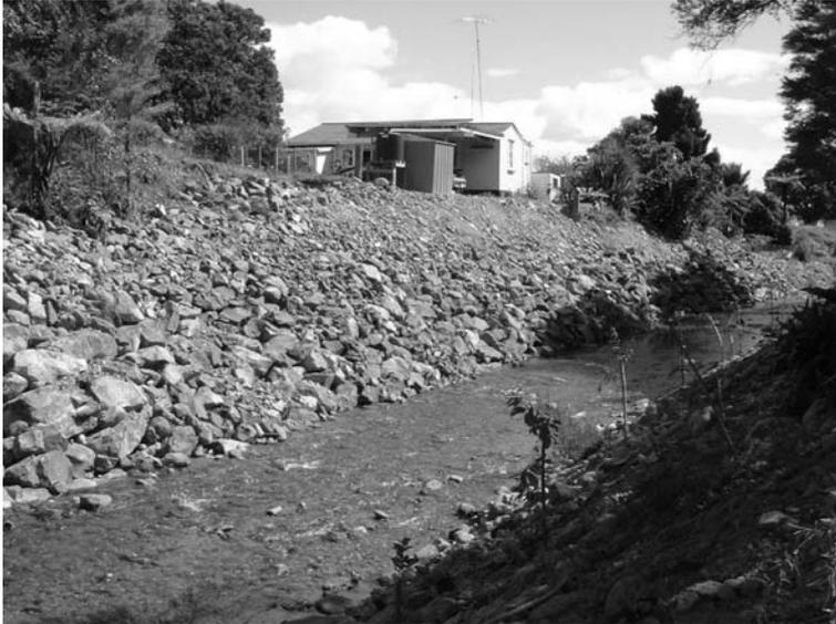
*Figure: Erosion control works in the Waiomu Stream*
