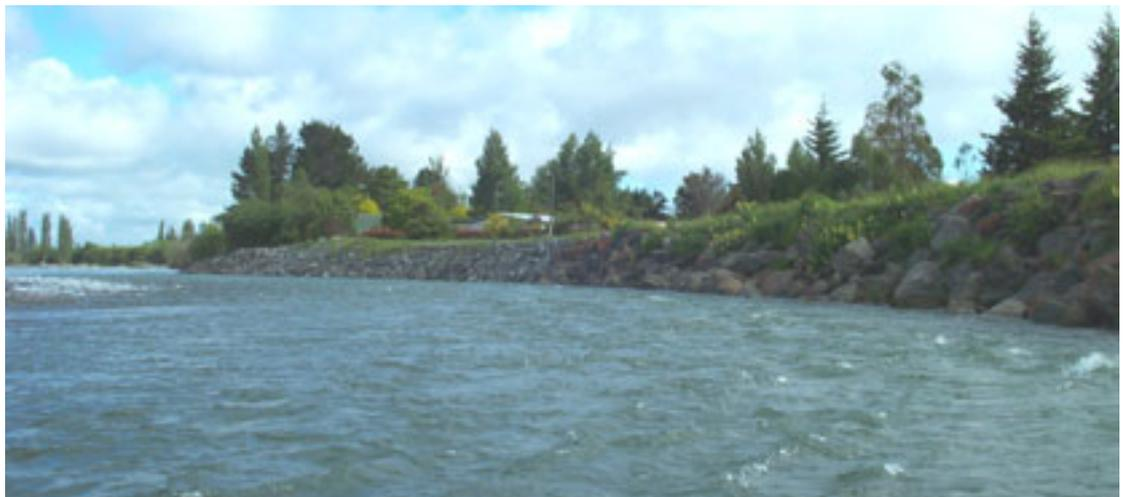
**Figure 11: Rock to protect Herekieke St Stopbank from river attack.**
