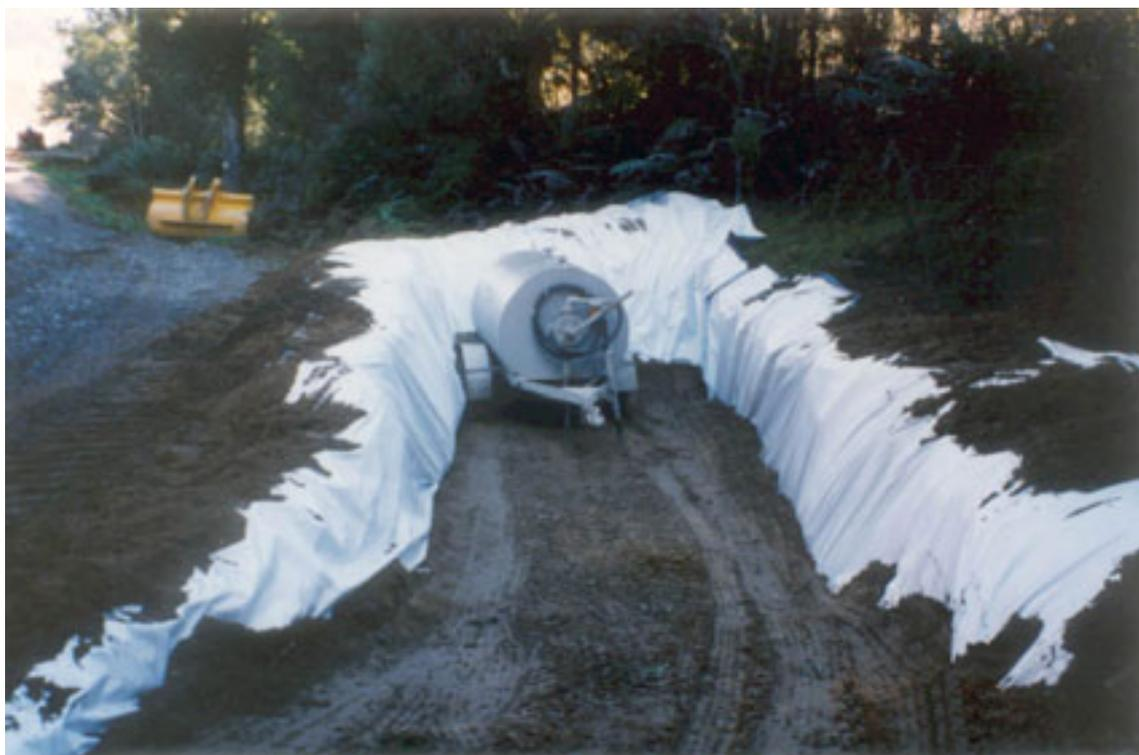
**Photo 1 Designated refuelling area contained by an earth bund and lined with impermeable plastic.**
