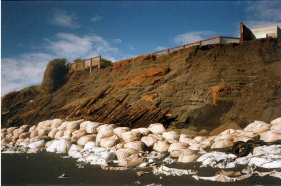
**Figure 2: Protection Work on Eroding Properties at Mokau Spit (Environment Waikato)**
