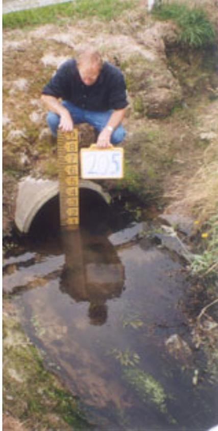
Figure 5 Culvert considered to restrict fish passage at high flows (culvert barrel is over half full at normal flows)
