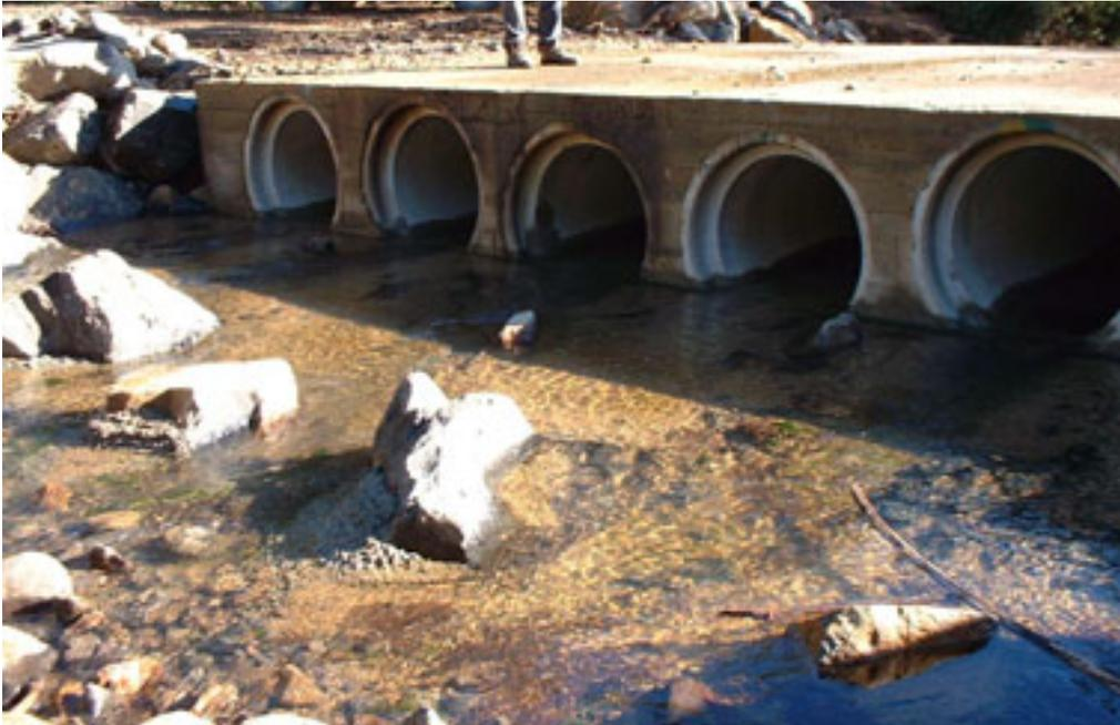
Figure 3 Culverted ford with none or minimal restriction to fish passage - culvert barrels are offset at different heights to allow for changes in flow
