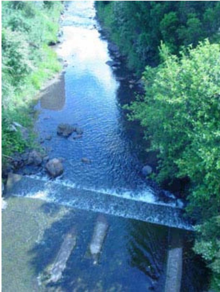
**Figure 3.1:** The concrete apron below State Highway 25 bridge could be a barrier to the upstream migration of torrentfish and inanga, and may explain why none were caught in the upland reach.
