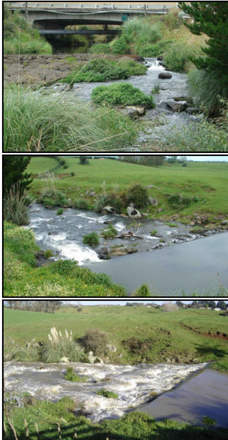
**Figure 2.2:** A weir was installed to improve the accuracy of the flow recorder at State Highway 22. The entire flow passes over the V-notch metal weir at lower flows (upper picture view upstream 17/1/2007, flow 0.27 m<sup>3</sup>/s), with higher flows spilling over the full width of the concrete-lip (middle picture looking downstream 26/10/2006, flow 1.02 m<sup>3</sup>/s, lower picture 2/07/2007 flow 5.4 m<sup>3</sup>/s).
