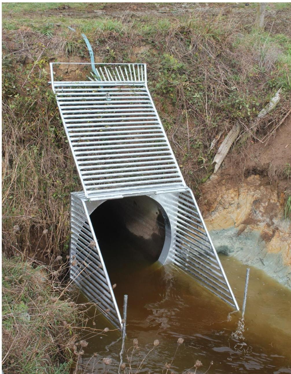
**Figure 1.** Installation of the Lake Ohinewai one-way koi carp barrier on the downstream side of the culvert running under Tahuna Road in May 2011. The barrier was designed to allow fish passage downstream out of the lake, but prevent upstream movement of adult koi carp.
